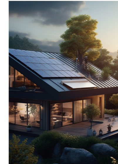
Residential Photovoltaic Energy Storage
