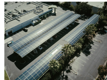
Photovoltaic Energy Storage and Charging Station
